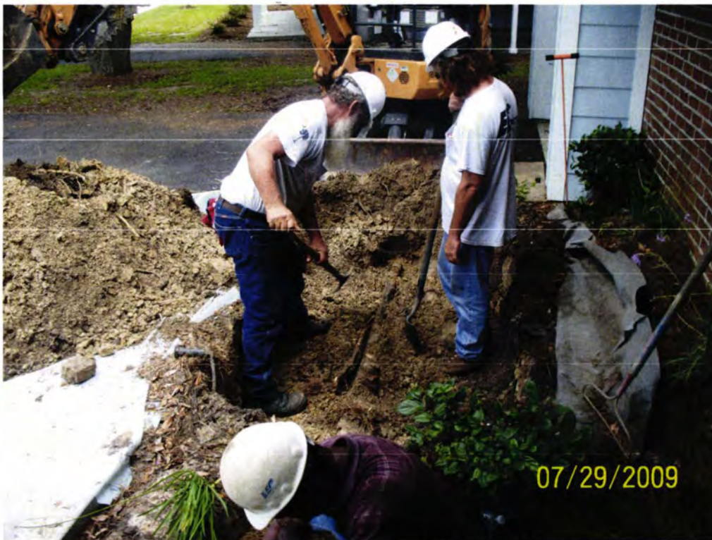
Picture 1: Sewer line is being temporarily removed before continuing with UST 1412Eagle excavation.
